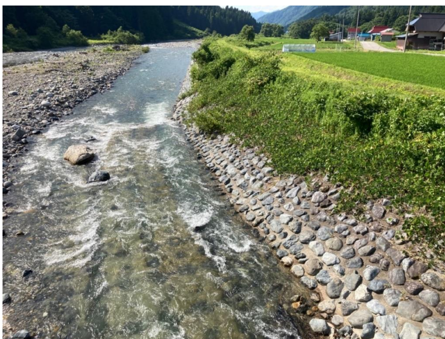
Photo 4-8 A revetment constructed during the river improvement after the Niigata and Fukushima heavy rainfall disaster in July 2011 (right bank, Kuratani). Local natural stones were embedded in the revetment to harmonize it with the surrounding landscape, but as a result, loose stones on the river bed, which provide habitat for freshwater fish and other species, were lost. In order to promote inland water fisheries that utilise the forces of nature to be described in 5.5-(7), river management that conserves an environment suitable for freshwater fish habitat.
