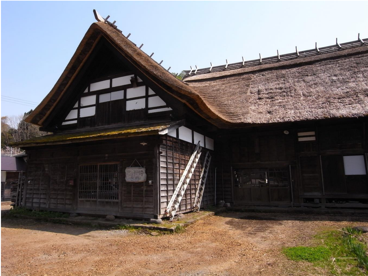
Photo 6-20 “Residence of the Hasebe Family (Kanozu guardhouse site)” managed and opened to the public by the Education Board of Tadami Town
