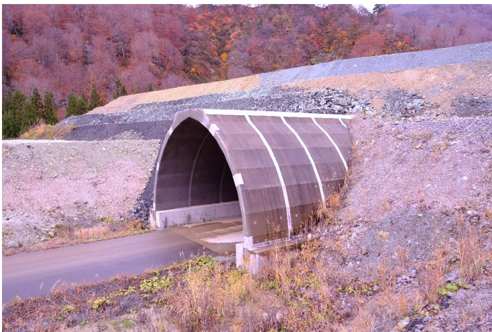
Photo 4-5 Place for soil from tunnel excavation. Revegetation by planting Japanese beeches ( Fagus crenata ) from other areas was planned, but the Tadami Biosphere Reserve Contributing Board has proposed to prevent soil runoff by making the slope gentler and to use natural vegetation succession for revegetation.
