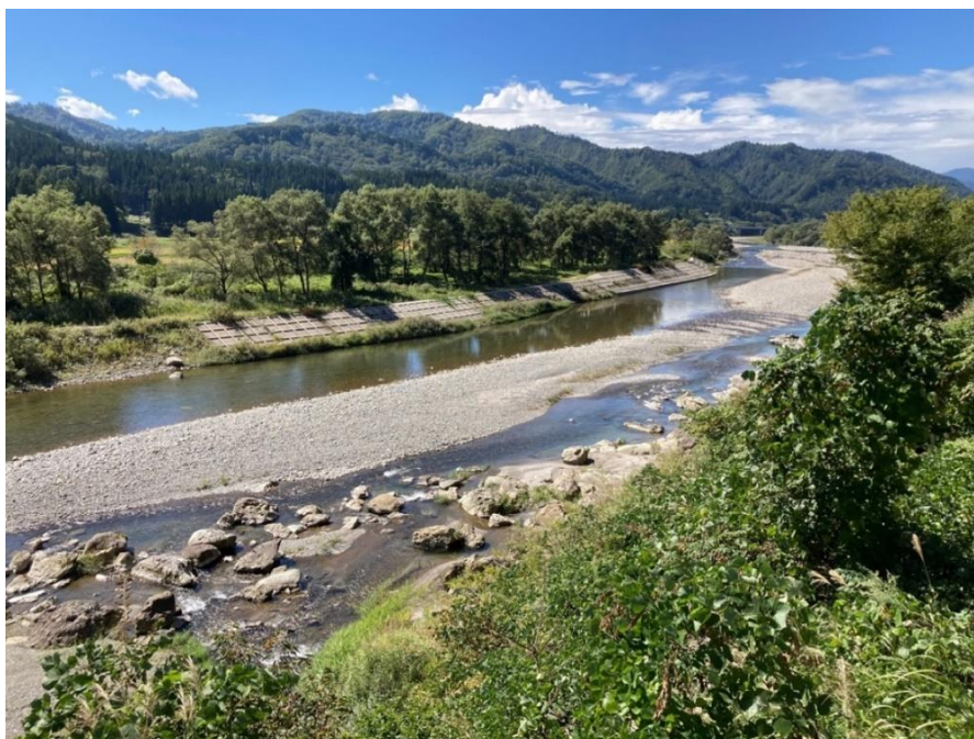
Photo 4-7 A new bank was constructed outside the existing bank during the river improvement after the Niigata and Fukushima heavy rainfall disaster in July 2011 (left bank, Okura). A riparian forest including S. hukaoana is confined within the bank, which is not affected by river disturbance. Since S. hukaoana depends on the river disturbance system for renewal, it is thought that the population here will be difficult to renew and will decay.
