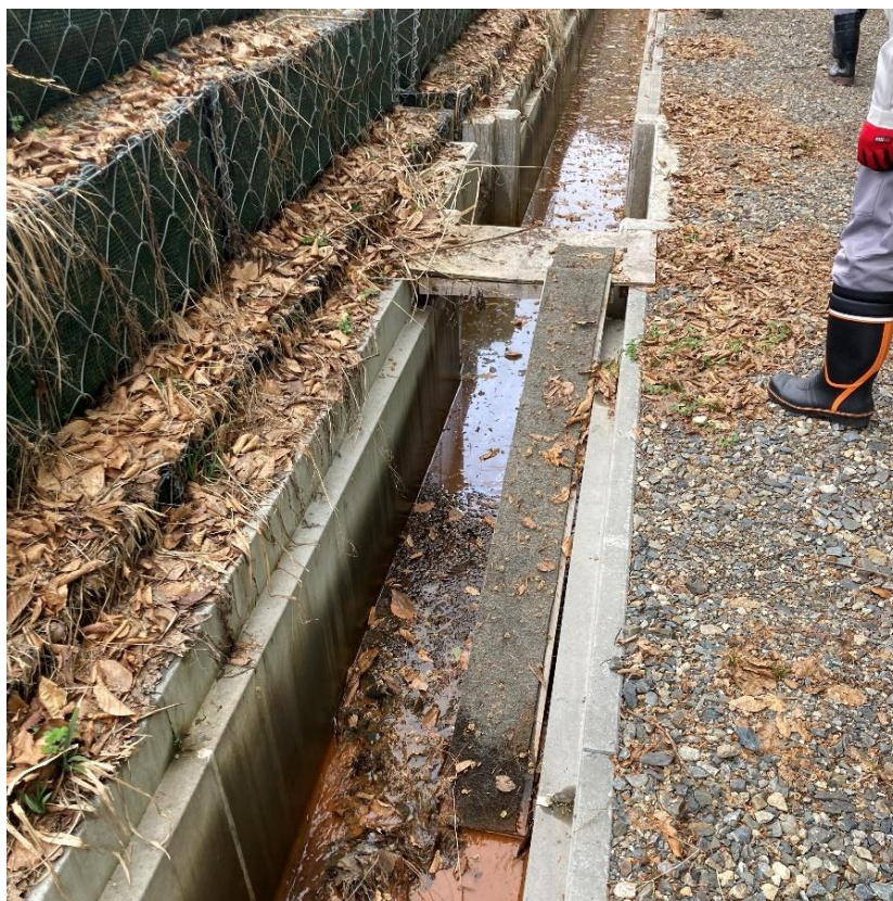
Photo 4-11 A ramp installed by Electric Power Development Co., Ltd. for small animals to crawl out of a gutter
